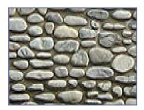
Normally you would take a trailer or small truck to collect river stone greywacke. When you are walking around selecting, keep in mind that you will be building a wide bed for the wall so that it is stable, and that you will need a variety of rock sizes for strength, gap filling and as capstones, so you can construct the style that is planned for the wall.
